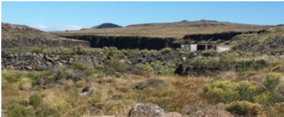
View of Dam Site and Diversion Gate (Photo by Molly Pitts).
